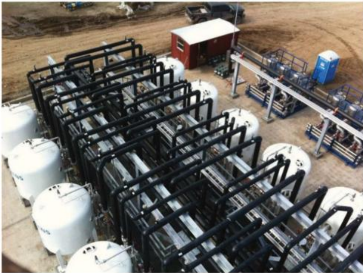
FABRICATED SPOOLS - Prefabricated HDPE Spool pieces installed for well injection treatment
