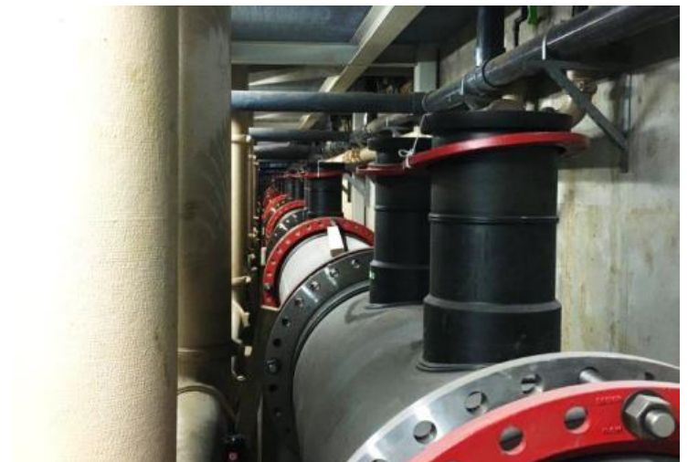
FRESHWATER FILTRATION PIPING SYSTEM - USF fabricated and installed 42" – 12" HDPE pipe.
