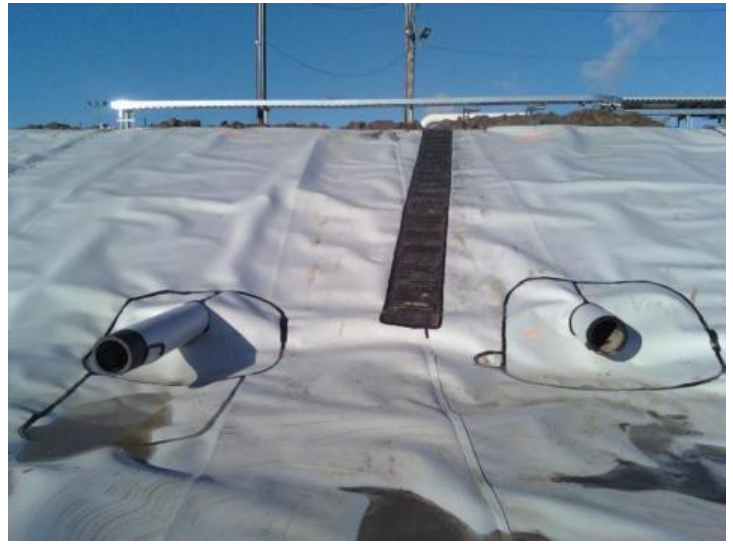
BRINE POND CONTAINMENT – 3 layer 80 mil black/white conductive liner installed by US FUSION.
