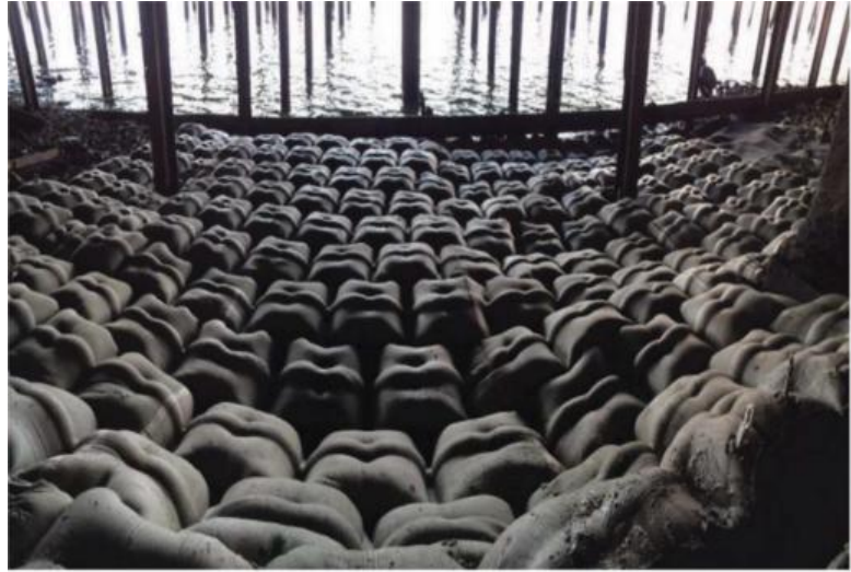
EROSION CONTROL USF installed 8" thick articulating block concrete mattresses for erosion control beneath a wharf along the Mississippi River. USF crews were able to install the revetment by attaching to retaining wall on one end and running product out, extending into river. Project was custom fitted to install around deck piles and columns.
