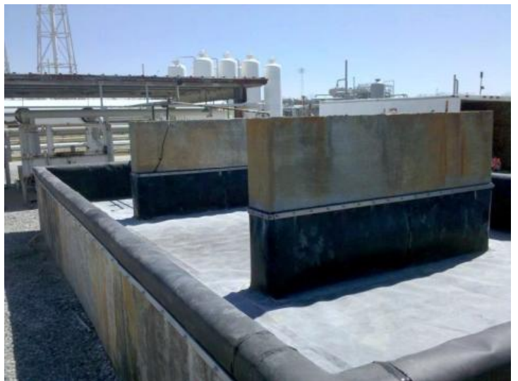
SECONDARY CONTAINMENT – Installation of PVDF liner as secondary containment in a petrochemical facility.
