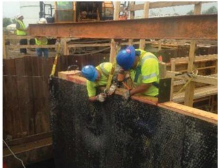
CONCRETE PROTECTIVE LINER – USF installed HDPE concrete protective liner onto formwork for acid neutralization sump construction.
