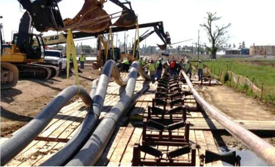
UTILITY PIPING - 2,600 LF of various size HDPE Pipe HDD drilled under a state highway. Installed, fused, tested & pigged by USF.
